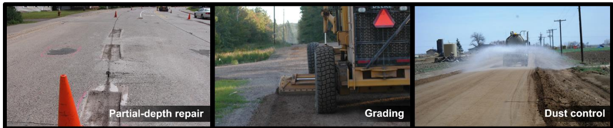
Figure 6: Examples of capital preventive maintenance treatments, cont'd—(from left) concrete road prepared for partial-depth repair, gravel road undergoing maintenance grading, and gravel road receiving dust control application (dust control photo courtesy of Weld County, Colorado, weldgov.com).
