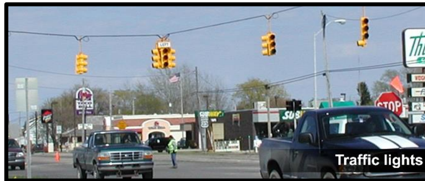
Figure D-1: Example of traffic signals
