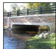
Figure 4: Three-sided box bridge
